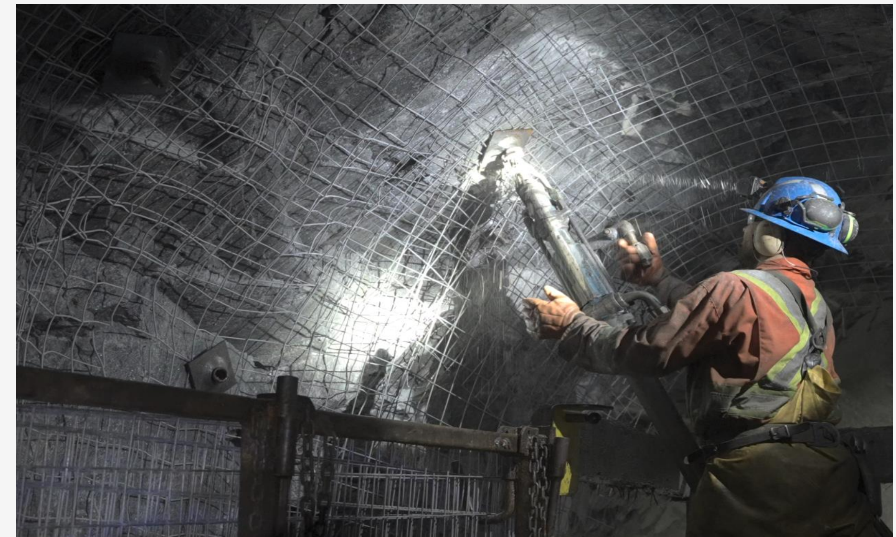
Bolting and meshing - July 2022
